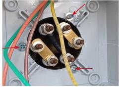
4. Remove the screws from the plastic enclosure that are connecting it to the heating element. The ground connection will require and allen wrench to remove.
