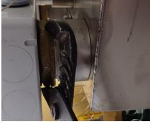
3. Carefully unscrew the heating element using the hex nut behind the plastic enclosure. If unable to easily access the hex nut follow Steps 4 and 5 to remove the plastic enclosure. If you are able to remove the element skip to Step 6.
