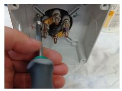
12. Remove the screws that are connecting the plastic enclosure to the heating element. The ground connection will require an allen wrench to remove.
