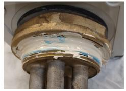
**9.** Apply TFE paste over tape & thread. Ready to install.
