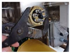
Carefully unscrew and remove the heating element using a pipe wrench or channel lock.
