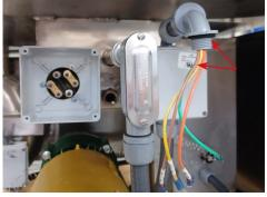
2. Remove lid and take a photo of the electrical connections to reference later. Disconnect the electrical connections and carefully move conduit.
