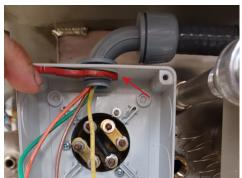
**16.** Feed the electrical wires and secure the conduit to the plastic enclosure.
