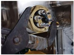
**13.** Carefully start by hand to screw the heating element into the tank. Do not tighten all the way until the plastic enclosure is attached to the element.
