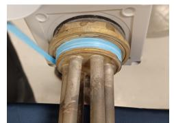
**8.** Apply Teflon Tape, leaving lead thread open to reduce cross threading when reinstalling.
