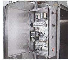
NEMA 4X CONTROL PANEL
